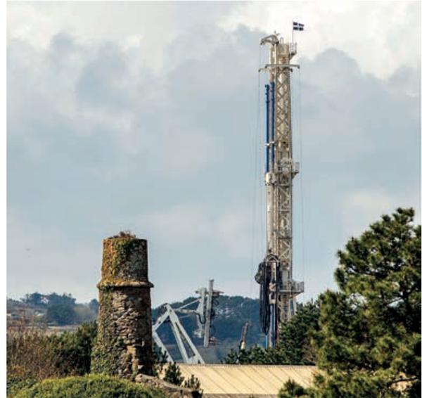
Temperatures in excess of 190°C have been measured in the wells. This natural heat source will be transferred from deep below the surface by water, which will be used to heat a binary power plant. Electricity will be generated 24 hours a day, delivering much needed baseload, which has a crucial role in an increasingly renewables-based grid. The potential for delivering renewable heat locally also begins to address the huge challenge of decarbonising the UK's heat requirement.
